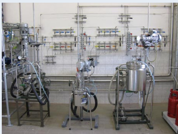
Figure 1: Autoclaves in the pilot plant of TITK applied for up-scaling of laboratory synthesis.
